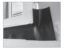
The first step is to apply two beads of adhesive to stick the preshaped EPDM sealing corners to the two bottom element corners on the wall and to the window frame. This can be done
